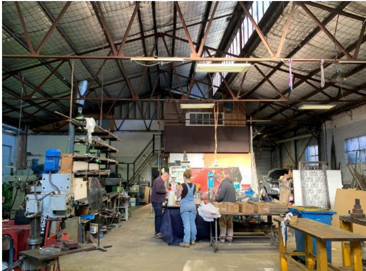
Figure 5: Interior view of the subject warehouse.
